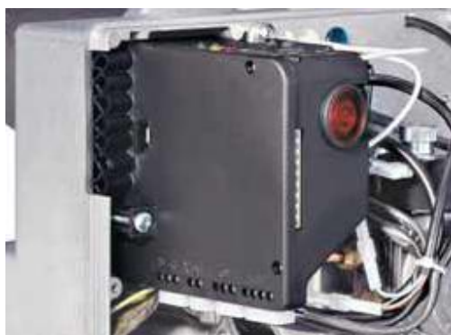
Control box fitted with ignition transformer
